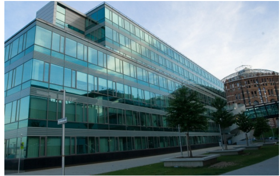
Office Campus Gasometer, Wien
