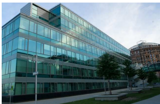
Office Campus Gasometer, Wien
